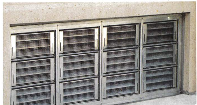
Engineered flood vents are part of a wet floodproofing strategy.
